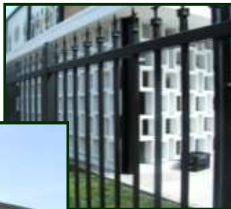
Right: Our new fence is 6ft tall with a decorative pointed top for added security.
